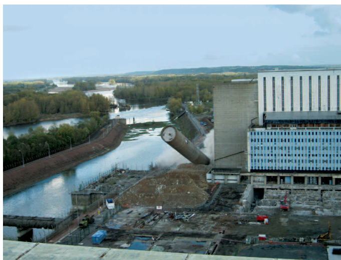
Chinon – blasting of the CHA 3 water tower
