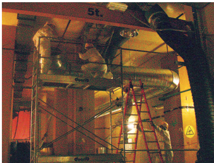
Brennilis – renovation of the ventilation system
