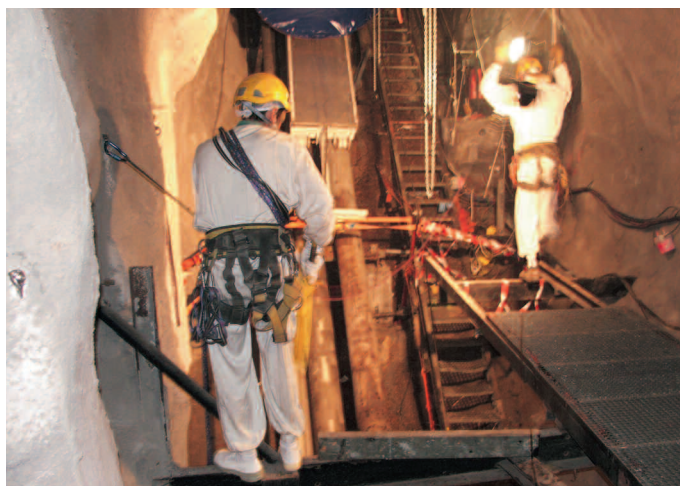
Chooz A – dismantling of ventilation flue
